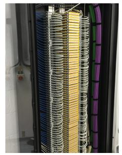
In total, 836 fibre optic cores were relocated to a new wall mounted splice enclosure (ODF) and 29 blown fibre tubes were either joined or relocated.
