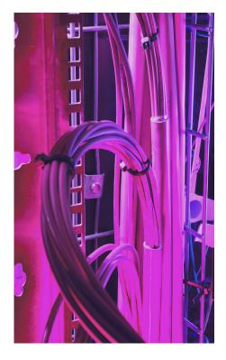
Sudlows engineers deployed over 6km of Blown Fibre tubes within the University's own existing ducting system.
